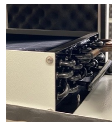
E-Coating on the heat exchanger circuit
